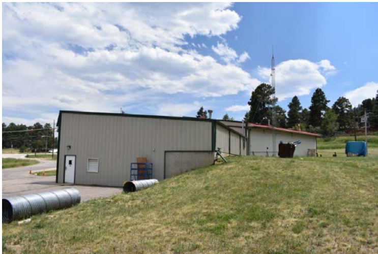
Picture #5.1 – Foundation wall north section, no concerns noted.
