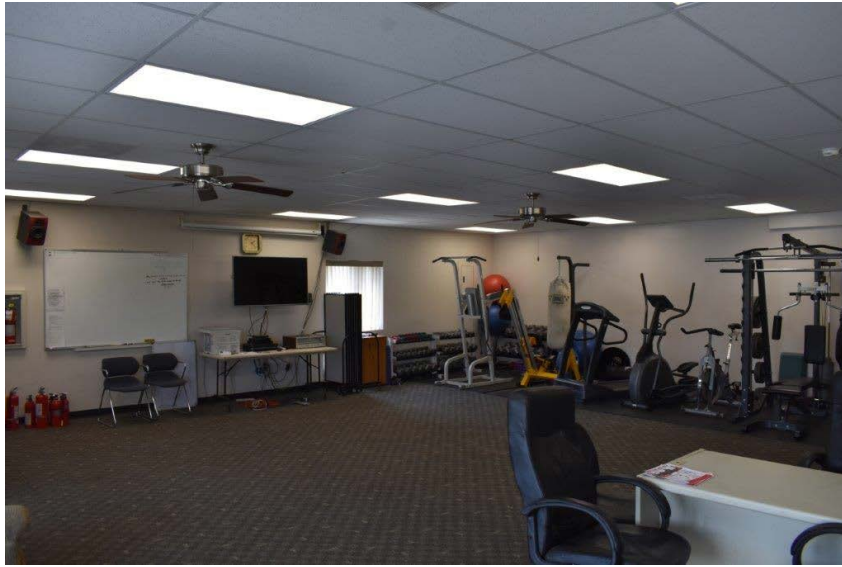
Picture 12.9 – Lighting in the administration wing is standard T8 lamped 2x4 troffers. It is recommended these be converted to LED fixtures.
