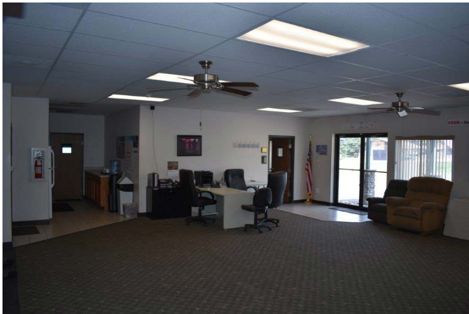
Picture #13.3 – Office area. No entrance vestibule, poor layout and use of space.
