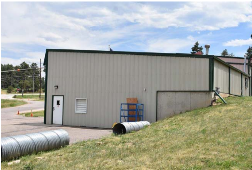
Picture #3.4 – The north side of the station.
