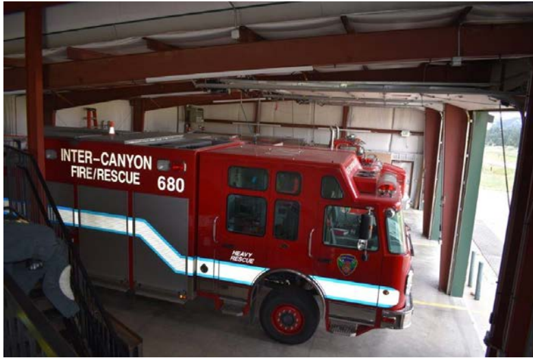
Picture #5.2 – General overview of the structural elements associated with the north section. No concerns.
