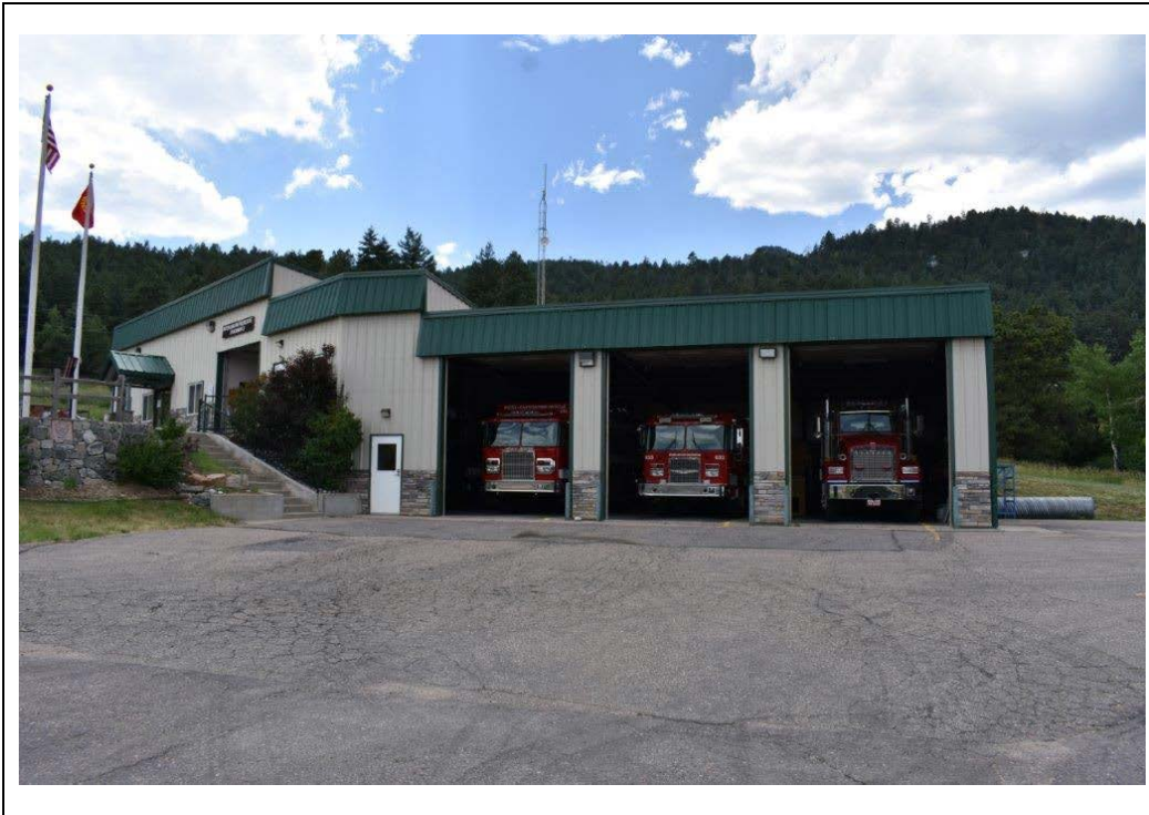
Picture #3.5 – The apparatus bay section. This is the newer side of the station, e.g., the north side.
