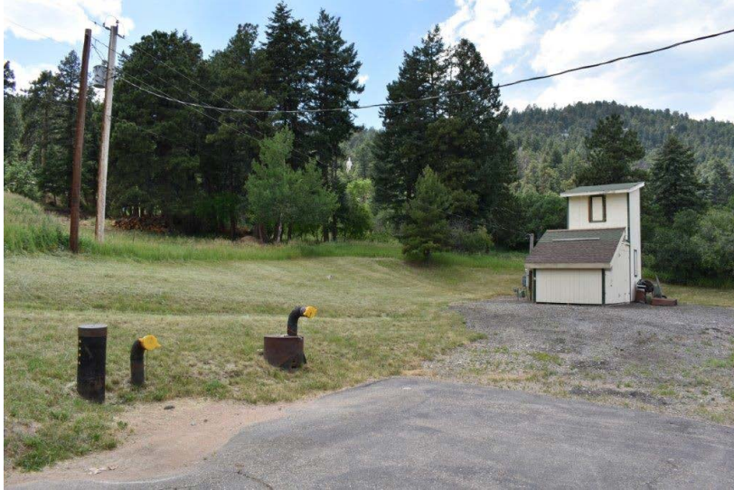
Picture #12.1 – Main service power pole.
