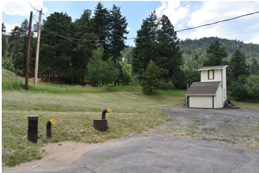
Picture #4.10 – This area represents the training prop area. Asphalt issues, grading issues, site should be paved or a suitable improved surface be installed.
