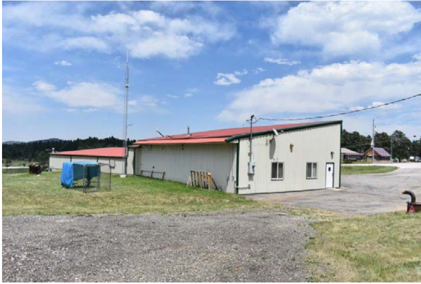
Picture #3.3 – the south and west side of the station. The lower roof section is the new “pre-engineered” section.
